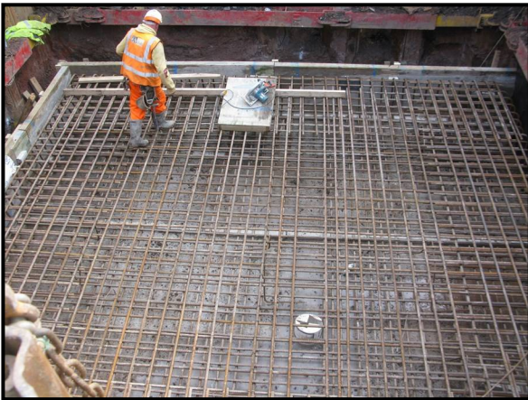
9. Reinforced concrete capping in base of Trench 1, from north.
