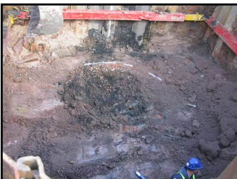
5. Base of Trench 1, showing Fill (110) and Mudstone (109), from south-west.
