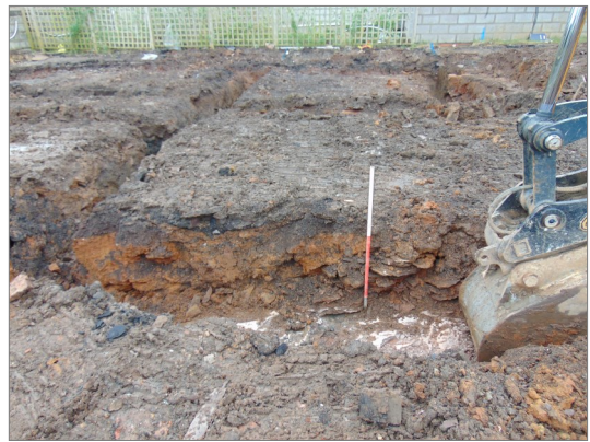
Plate 18 House 1 footings trench, bedrock is visibly high here. View south west.
