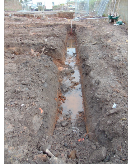
Plate 23 Foundation trench for house 3 view north east.
