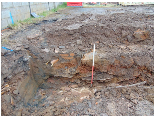
Plate 13 Brick built structure associated with tank and drainage system 118, seen in section of a foundation trench, looking south west.
