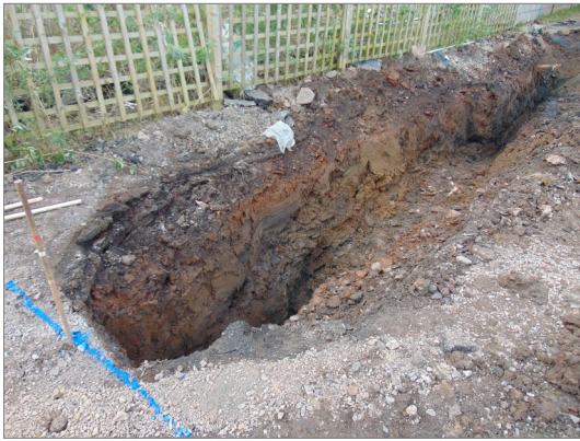
Plate 15 House 1 footings trench, view shows cut 116, looking south.
