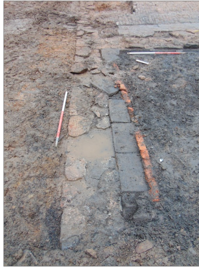
Plate 9 Rear wall 124, with abutting drain feature, 111, this section is edged with red bricks set on end. View north east.
