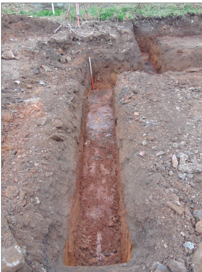
Plate 24 Foundation trench for house 3 garage view west.
