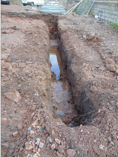
Plate 21 Foundation trench for house 3, view north east.
