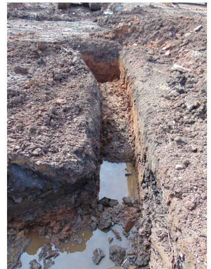
Plate 26 Foundation trench for House 2 where bedrock rises naturally. View west.
