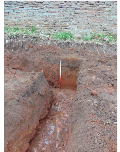
Plate 3 Foundation trench for house 4, view north east.
