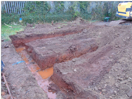
Plate 19 Foundation for house 1 garage, showing only sterile natural deposits, looking west.
