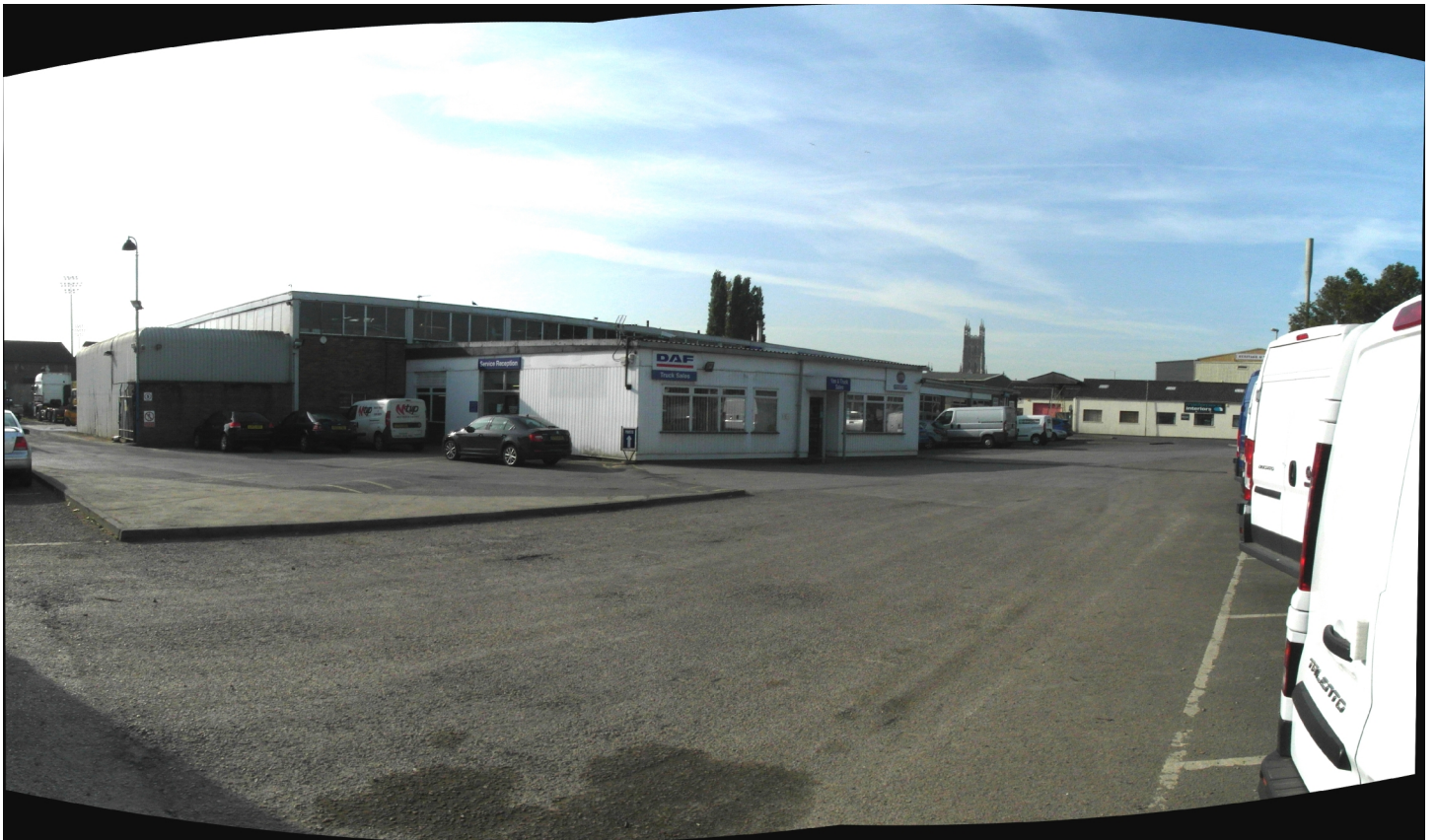
1. Composite panoramic view of the site, looking south-east on the left-hand side of the frame, to south on the right-hand side. The tower of Gloucester Cathedral can be seen in the background. This is the more northerly, and larger of the two buildings currently sitting within the site boundary. Both are modern and in terms of design, are of no architectural, historic or aesthetic interest or value.
