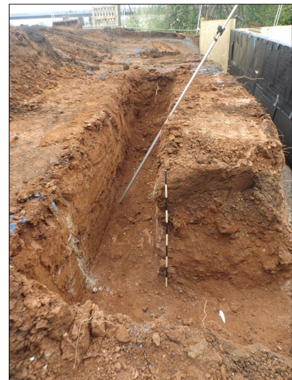
Plate 8: Foundation trenches cut through natural ground.
