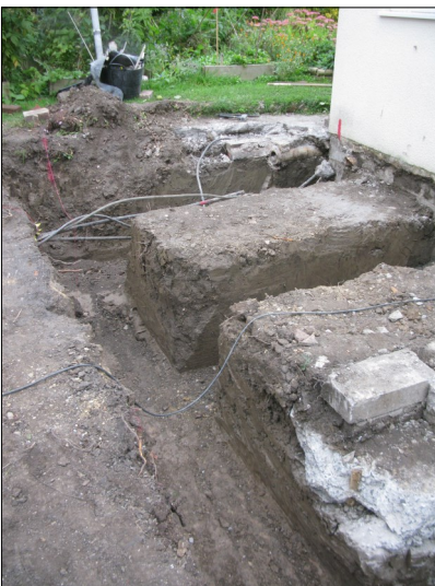
Plate 3 General view of the foundation trenches looking east.
