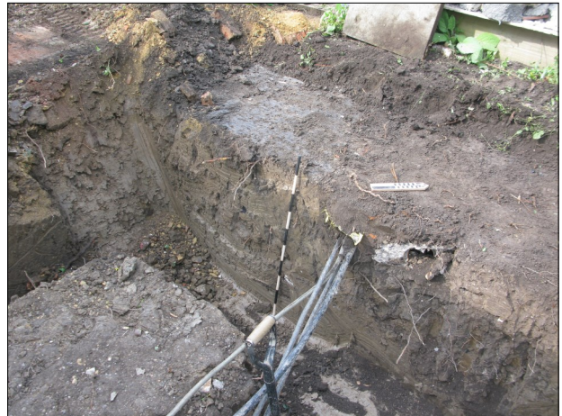
Plate 2 General view to north-west showing a number of service cables extending from the section. The cables are within a shallow trench which cuts a natural subsoil layer.
