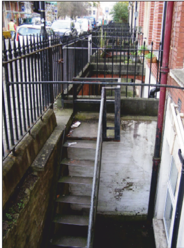
37. Frontage of surviving historic terraces in Cave Street, immediately to the south-west of the development site, showing arrangement of lower ground floor rooms accessed by steps from street level, and descending to a small, paved yard. This is the same arrangement that existed historically in the terraces fronting the south-western side of Dean Street. The steps here are obviously modern.
