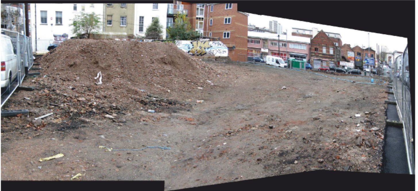
1. Composite general panoramic view of the site, prior to the excavation of the first phase of test pits. Taken from the south-eastern corner of the site, close to the junction of Dean Street and Chapter Street. The view pans round from south-west on the left-hand side of the frame, to north-west on the right.
