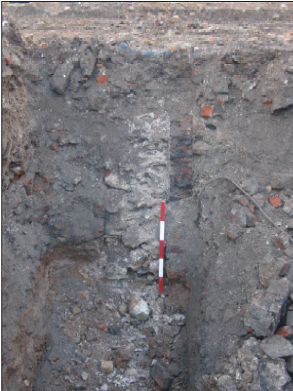
25. PP 14, wall, context 1401, view to north-east. Attached brick wall against south-eastern elevation. Scale: 1m
