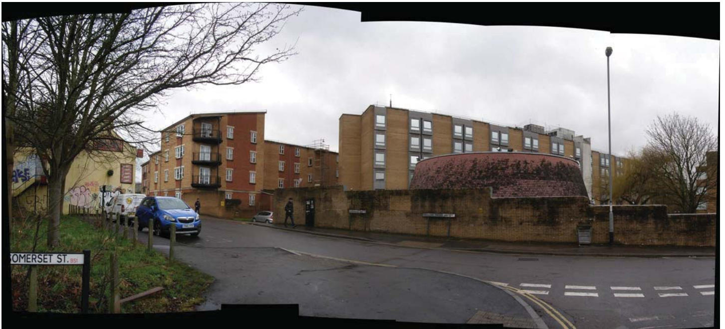
1. Composite panoramic view close to the junction of Somerset Street and Prewett Street. The shot pans round from roughly west on the left hand side of the frame, to north on the right hand side. The Grade II listed glass cone appears centre right, and the Bell Inn building, earmarked for removal, on the left. The proposed new main residential block will rise massively above the viewer at the left hand side of this shot.
