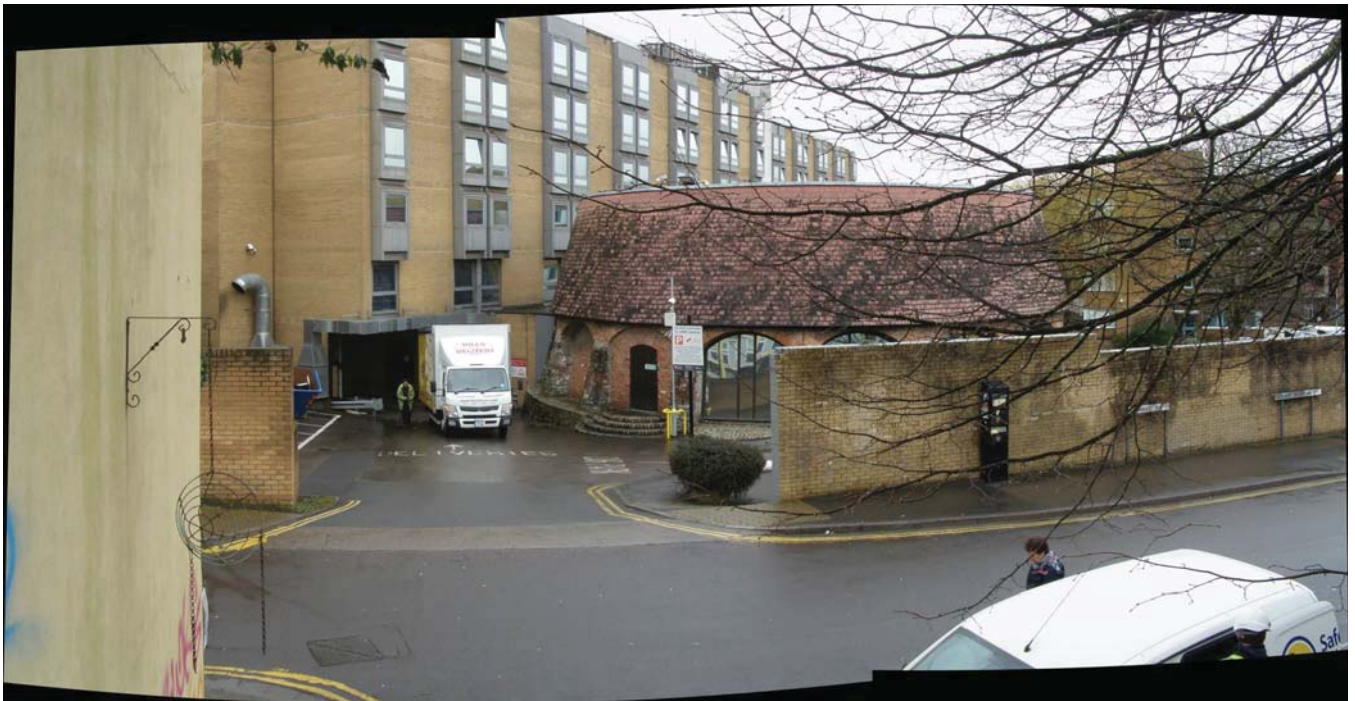
2. Composite panoramic detail of the listed glass cone, looking north. The north-eastern elevation of the Bell Inn appears on the left of the frame. From the street, the cone is partially obscured by the car park wall
