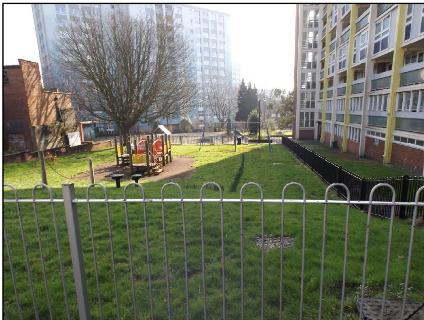
4. View to south-east into the upper grassed playground area fronting onto the south-eastern side of Prewett Street, immediately south-west of the two extant historic buildings. The north-eastern elevation of Proctor House on right. The boundary of the new development runs north-west/south-east a few metres in front of Proctor House.
