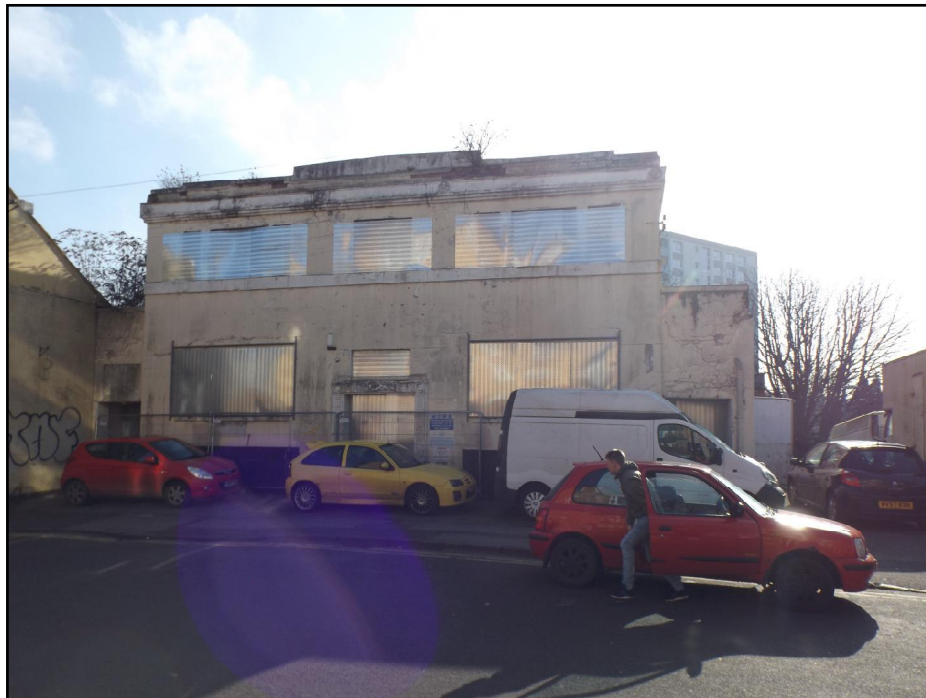
2. Redcliff Adult School, detail of frontage. View to south-east.
