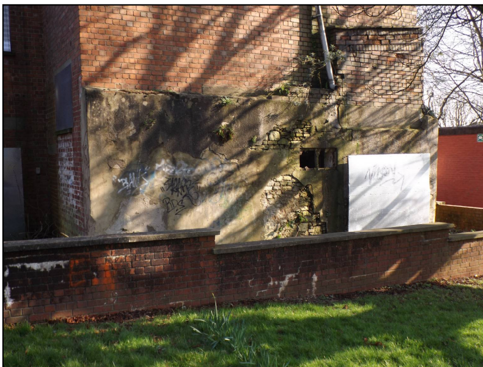
6. Detail of the wall shown in its wider context in Plate 5 . The lower part is clearly historic masonry fabric, and with the exception of the two standing historic buildings, it seems to be the only small remnant on the entire site of the buildings and structures which once covered it.
