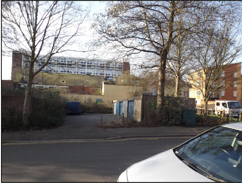
3. View from Somerset Street looking south-west. Residents' garages in foreground, the north-eastern elevation of The Bell Inn just beyond. In the background, the roof of the former Redcliff Adult School shows considerable damage. The north-eastern elevation of Proctor House towers above the Adult School building.
