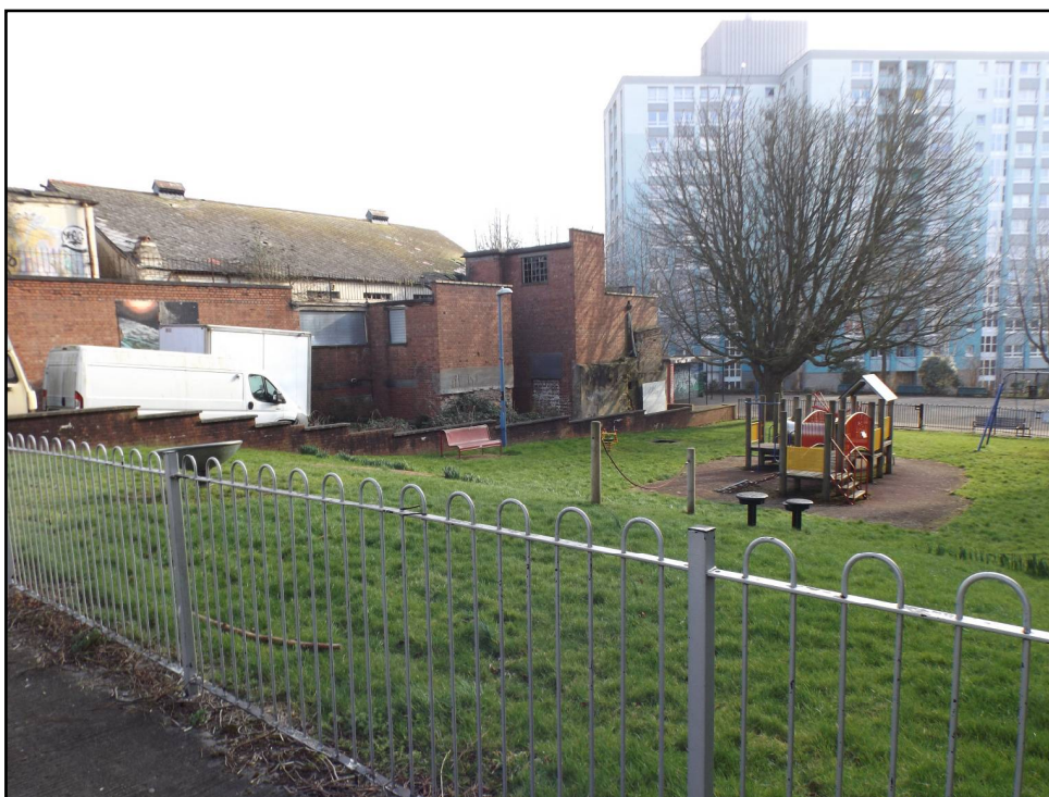
5. General view to east from the south-eastern side of Prewett Street, towards the south-western corner of the Redcliff Adult School Building, onto which later (post WW2) brick extensions have been butted.
