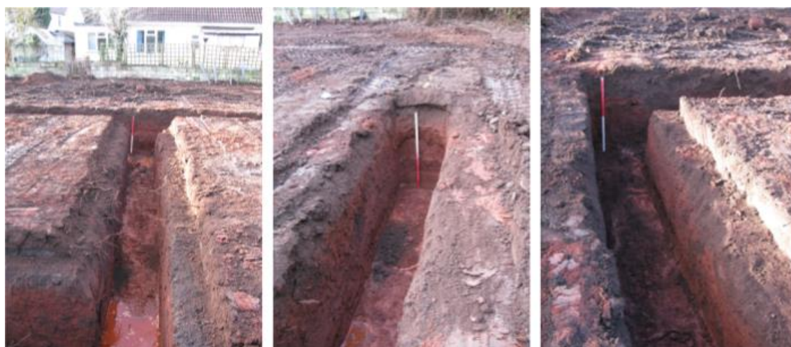
Plate 1: Shows excavated foundation trenches
