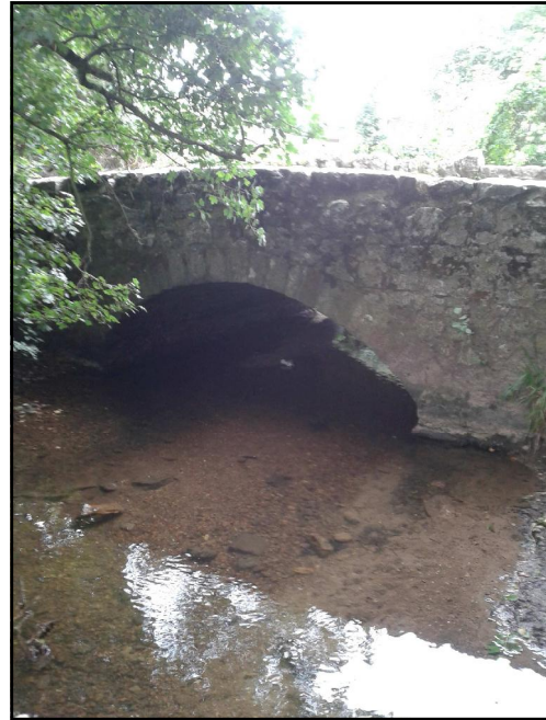
2 Kate Bridge, view approximately to north.
