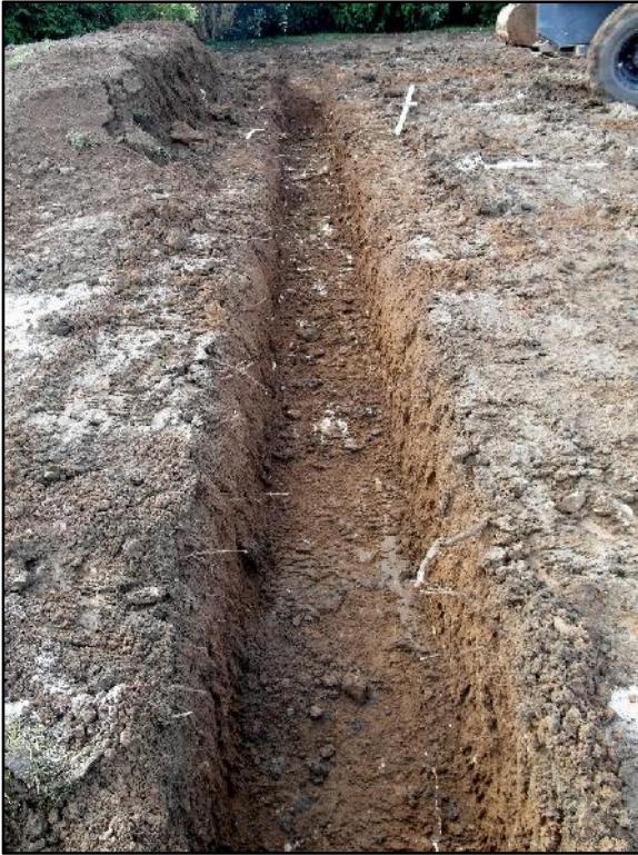
8. Trench 2 of House 3 complete (see Figure 3 ). View to north-west.
