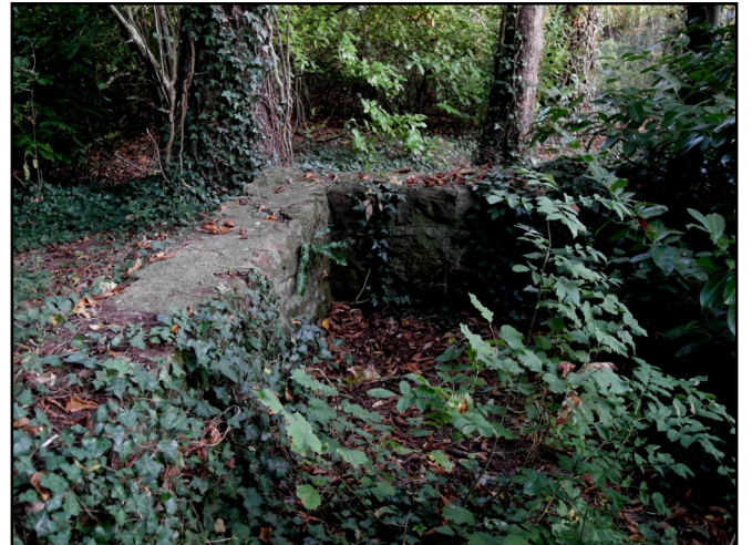
3. View of the north-west corner of the masonry structure in woodland and undergrowth on the western side of the Lydeard road, and immediately to the north of Cotford Bridge. It is marked on OS maps from the end of the 1920s, but its function when in use is, at present, entirely unknown. It lies within the site boundary, at its extreme south-eastern corner.
