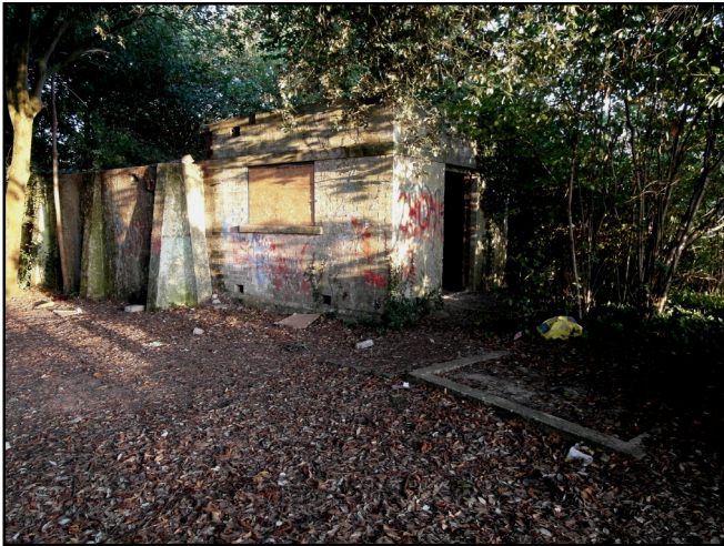
2. The group of structures at the north-eastern side of the site identified as 'tanks' on modern OS mapping. View to north-west.
