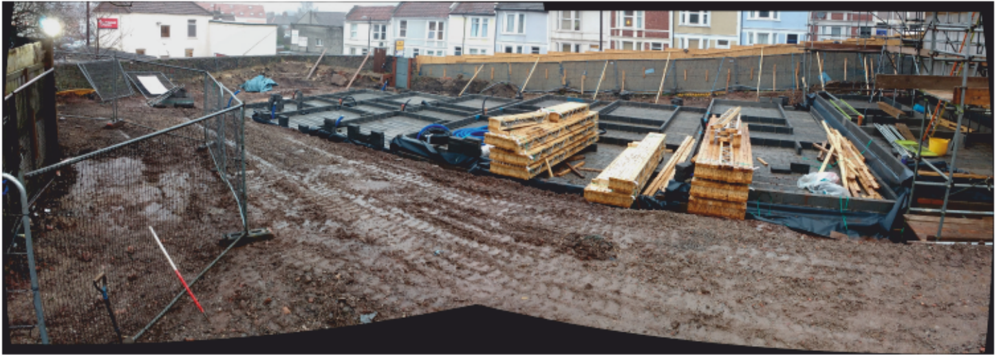
4. Composite panorama of the south-western part of the site, prior to investigations in the extreme south-western corner. The trenches shown in Plate 3, in the centre of the frame, have now been concreted, and construction of blockwork has commenced. The view pans round from south-west on the left-hand side, to north-west on the right-hand side. Houses lining the north-western side of Balfour Road are seen in the background.
