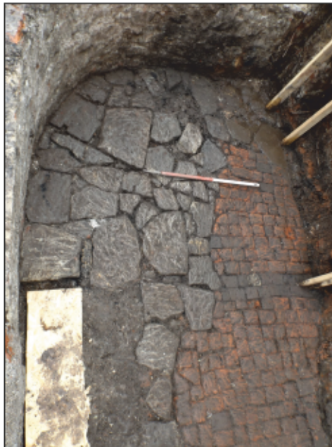
13. Detail of rough flagstone repair (110) to original brick sett flooring (105), at the south-eastern end of the building defined by wall (102), seen running down the left hand side of the frame. The bottom of secondary opening (106) through the main boundary wall can be seen framed by the wooden shoring at top right. Scale: 1m. View to south-east.
