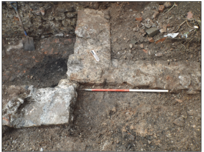
12. Detail of junction between wall (102) (left of frame), and (107) (top right quarter of frame). It became apparent that this junction had been badly truncated and in fact originally, probably represented a staggered T-shape all of one build. Scale: 1m. View to south-west.
