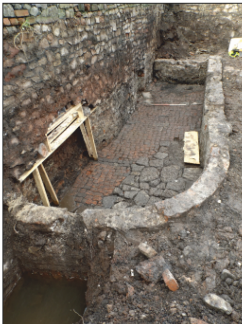
9. Wall (102) and, at the far end wall (107), returning south-westwards to butt against the main boundary wall, representing part of the same structure. The curve in the wall at the nearer (south-western) end of this building may be to accommodate a small wheeled vehicle turning in from the street, through opening (106) on the left. Scale: 1m. View to north-west.
