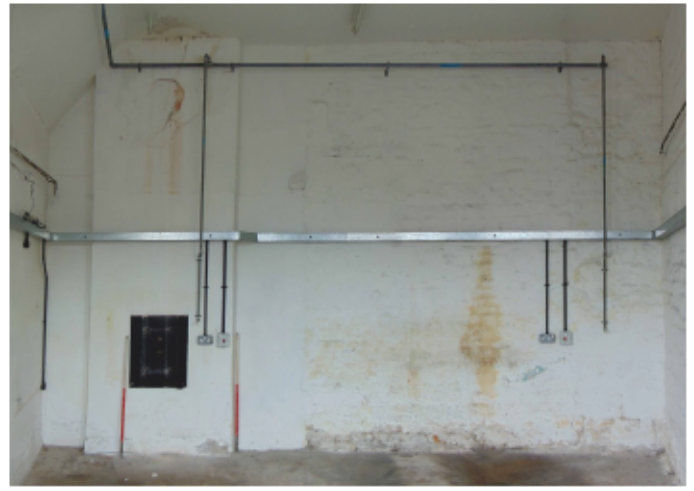
Plate 11: South facing ground floor internal elevation of office building.
