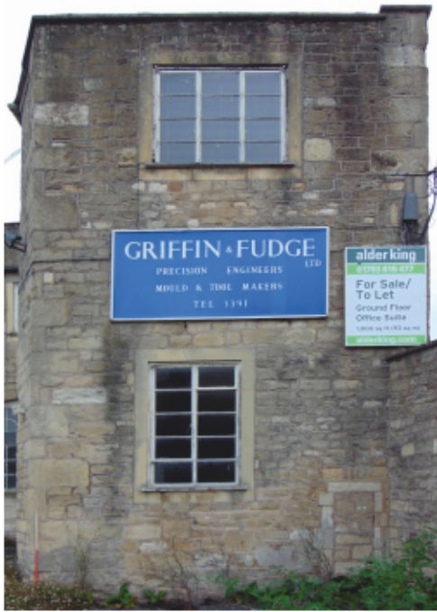
Plate 4: South facing ground floor external elevation of office building.
