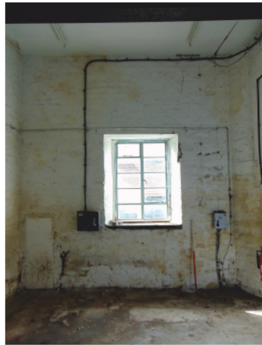
Plate 5: North facing ground floor internal elevation of office building.
