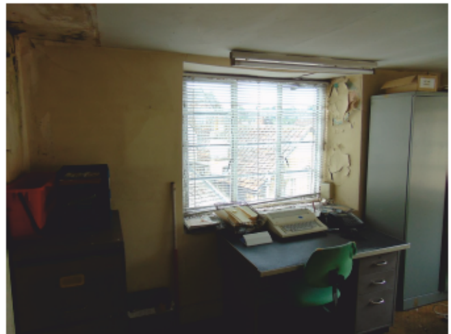
Plate 20: East facing first floor internal elevation of office building.
