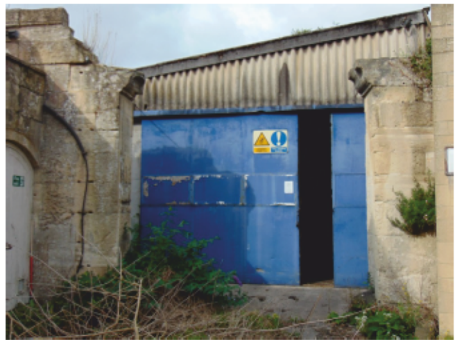
Plate 22: View through partially demolished 19th century arch to the southern range of the modern workshop building behind. Looking west.
