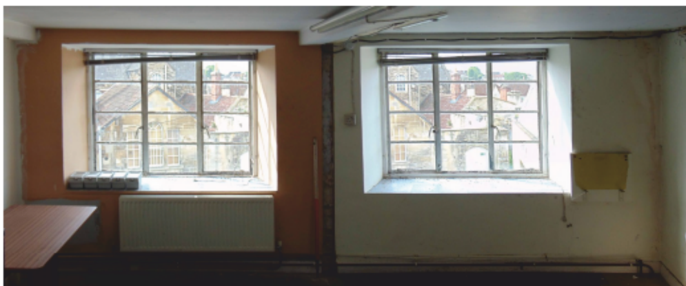
Plate 12: North facing first floor internal elevation of office building.
