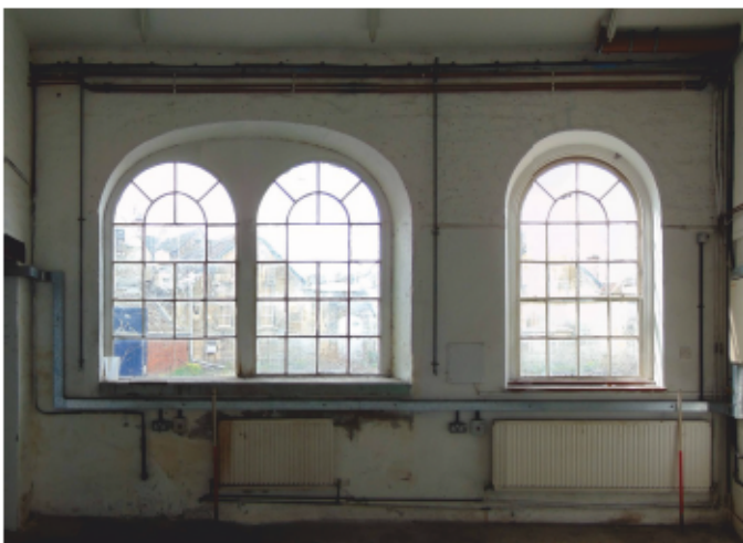
Plate 10: North facing ground floor internal elevation of office building.
