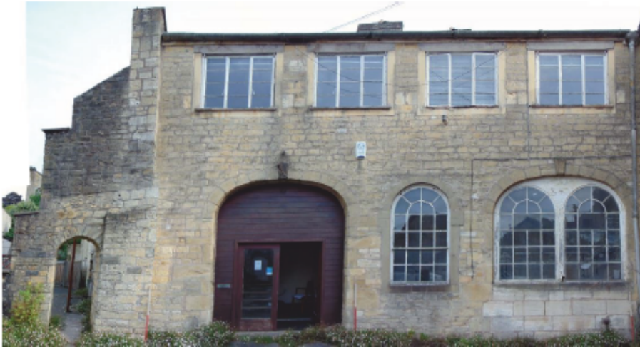
Plate 1: South facing external elevation of office building.
