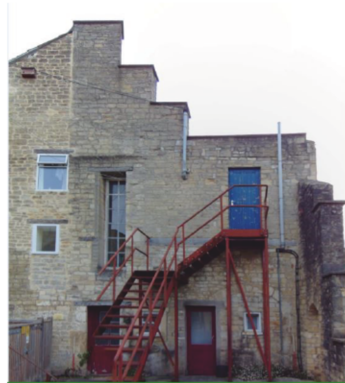
Plate 2: West facing external elevation of office building.
