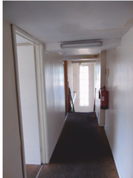
Plate 14: Looking west along first floor corridor of office building.
