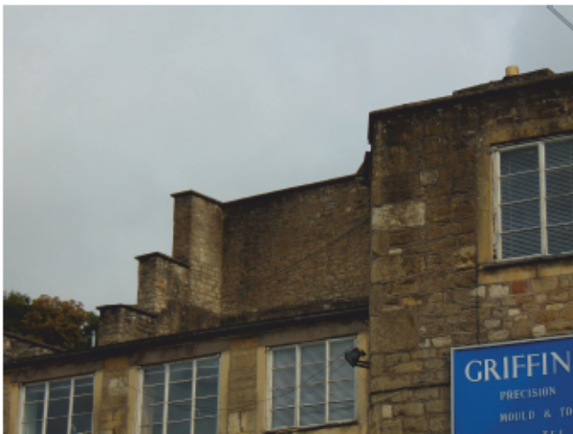
Plate 21: Looking north west at original roof line of office building.
