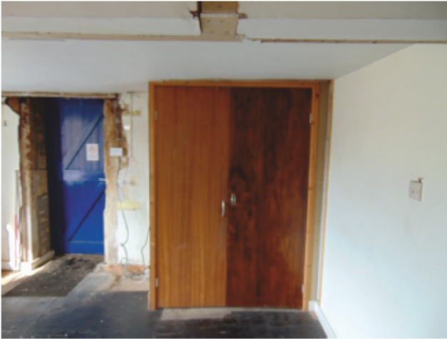
Plate 13: East facing first floor internal elevation of office building.
