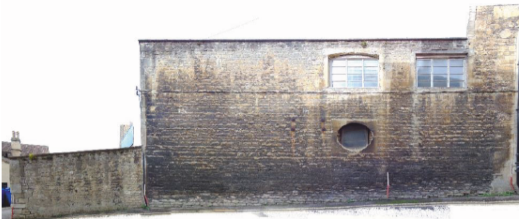
Plate 3: East facing external elevation of office building.
