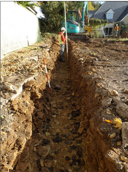
Plate 3. Looking north-east along the north foundation trench of the new building
