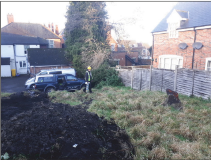
Plate 1: General view of site during trench excavation. Looking north west.
