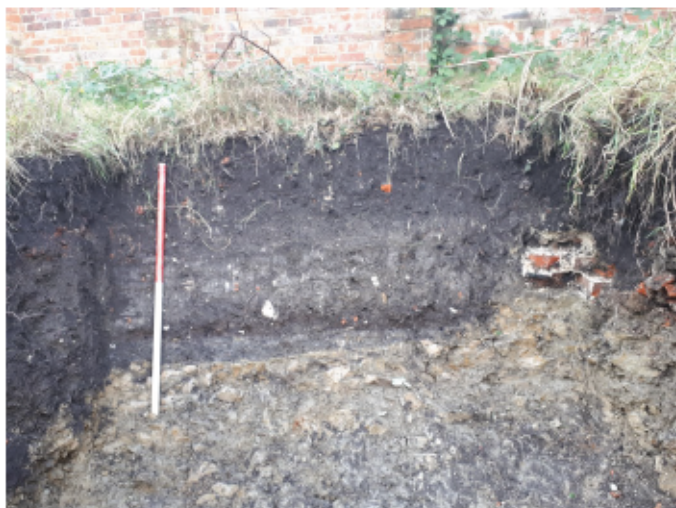
Plate 7: South west facing section of trench 2. Showing pit [204] to the left and wall 203 to the right. Buried soil 206 can be seen below wall 203 (see section 1). 1 x 1m scale.
