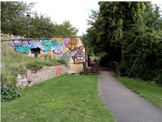
Plate 2. View along 'the northern boundary of the site, looking east.
