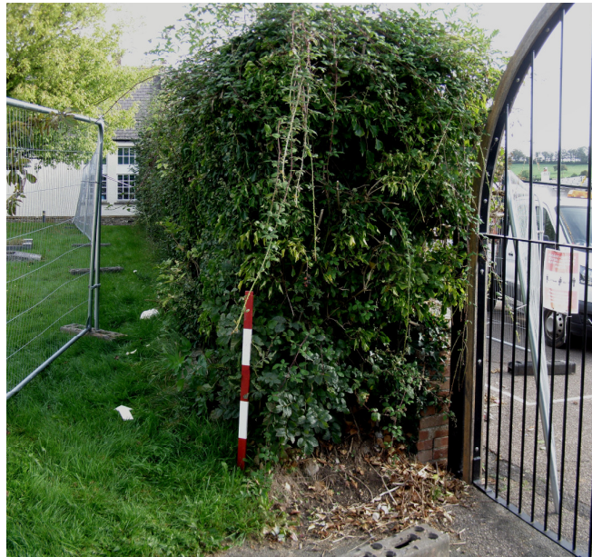
1. View along the hedgeline from its southern end, looking north, prior to the commencement of the work to remove it. The historic stone boundary wall within it is almost completely invisible, apart from a section of a later brick extension, acting as the northern jamb of the gate which leads from the school playground into the churchyard. Scale: 1m, view to north.
