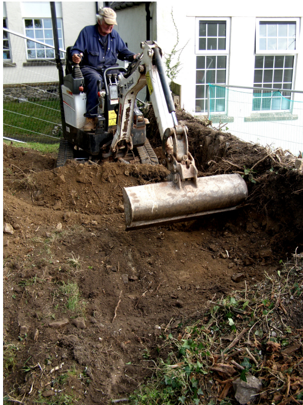
5. Following removal of the hedge, the bank which had supported it was levelled by machine.
