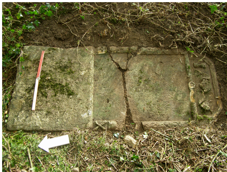
12. 18th century ledger slab (102). Note complete fracture across the width of the slab, resulting in extensive damage in the middle of the left-hand border. North as indicated, scale: 0.50m.
