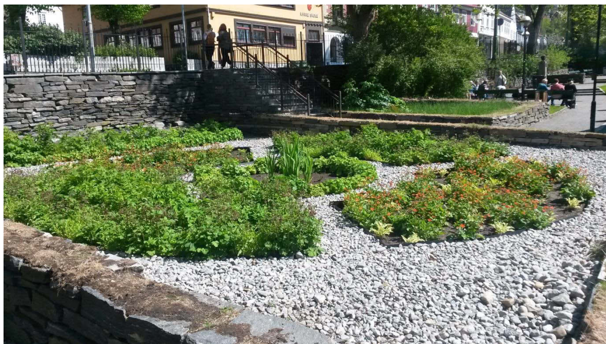
Figure 7 SUDS: Rainwater garden in Bryggen to help recharge waterlogged deposits
