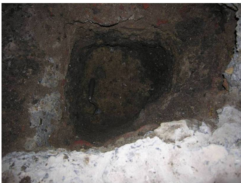
Photo 11 Sandy Concrete footing for existing basement at 0.9m bGL, looking south
