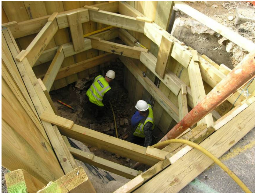
Photo 3 Western Access shaft, removing 19/20th-century building foundations and north–south aligned wall [20], looking south-east
