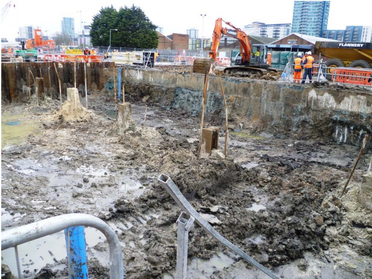
Photo 9 11kv electric cable route, where it crossed the main cut-and-cover tunnel
