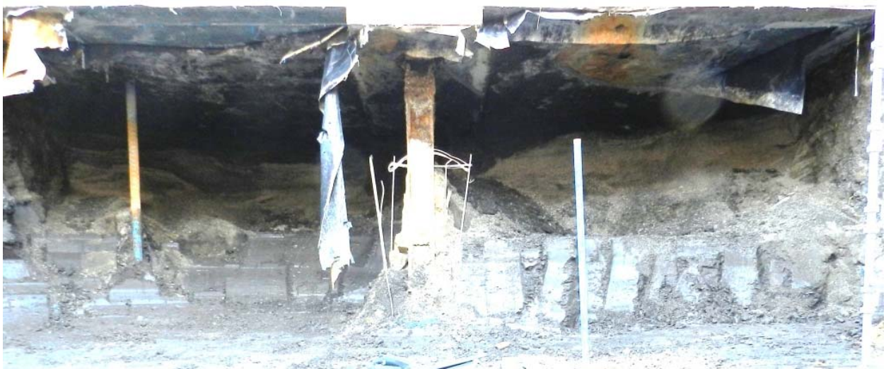
Photo 7 Terrace Gravel beneath the 11kv electric cable chamber, sedimentary structures indicate (potentially) a moving ice-age river channel. This contrasts with horizontal bedding observed elsewhere
