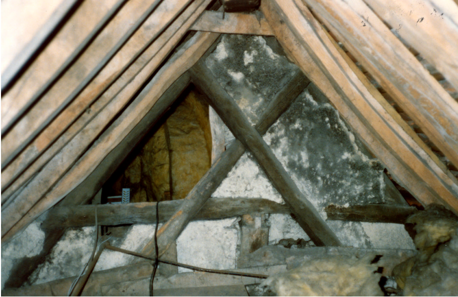
Fig. 5. The passing braces of truss T4a. The top of the inserted crown post and the severed collar plate can be seen below the collar, and the yoke and ridge of truss T4b are also visible.
