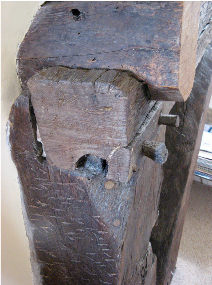
Fig. 7. Arcade post head, T3 (north). The tiebeam is a replacement, probably of the fifteenth century
