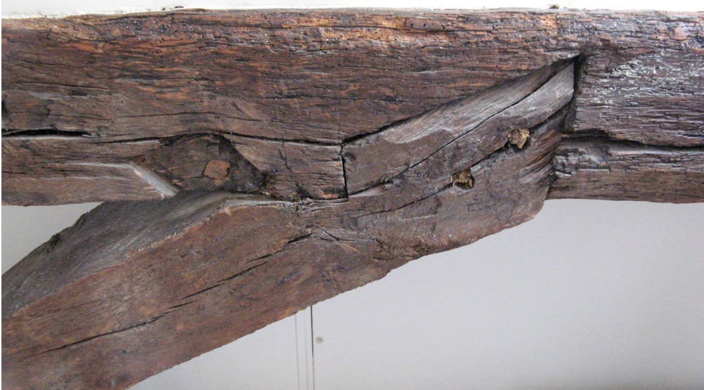
Fig. 6. Notched-lap joint with simple entry on the reused arcade plate, showing the matrix of a similar joint.
