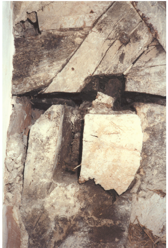
Fig. 8. Coggied joint of arcade plate, tiebeam and rafter (south side of truss T4a)
