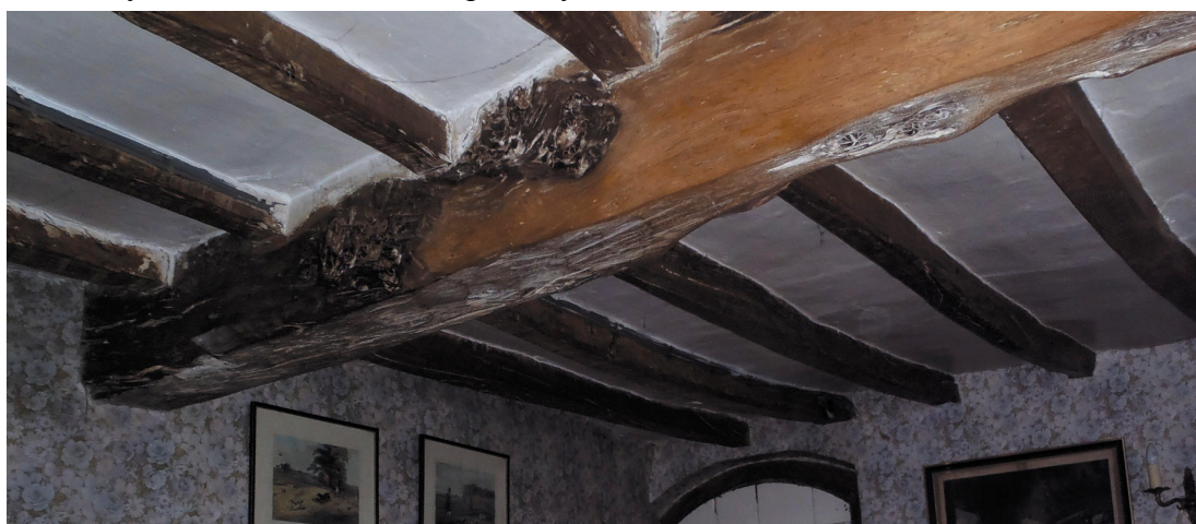
Fig. 4. The ceiling beam in bay III, showing the transition from the regular chamfered part to the waney end (Photo: Neil Finn).
