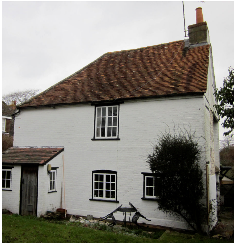
Fig. 1. Tibberton Cottage, Harwell, from the south (Photo: D. Clark)
