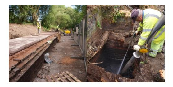
After cleaning, it turned out to be a simple drainage sump, with water from the platform and trackbed being fed into it. So, nothing very exciting, but a very tiny piece of information which somehow adds to our collective understanding. Such is the nature of most archaeology!
