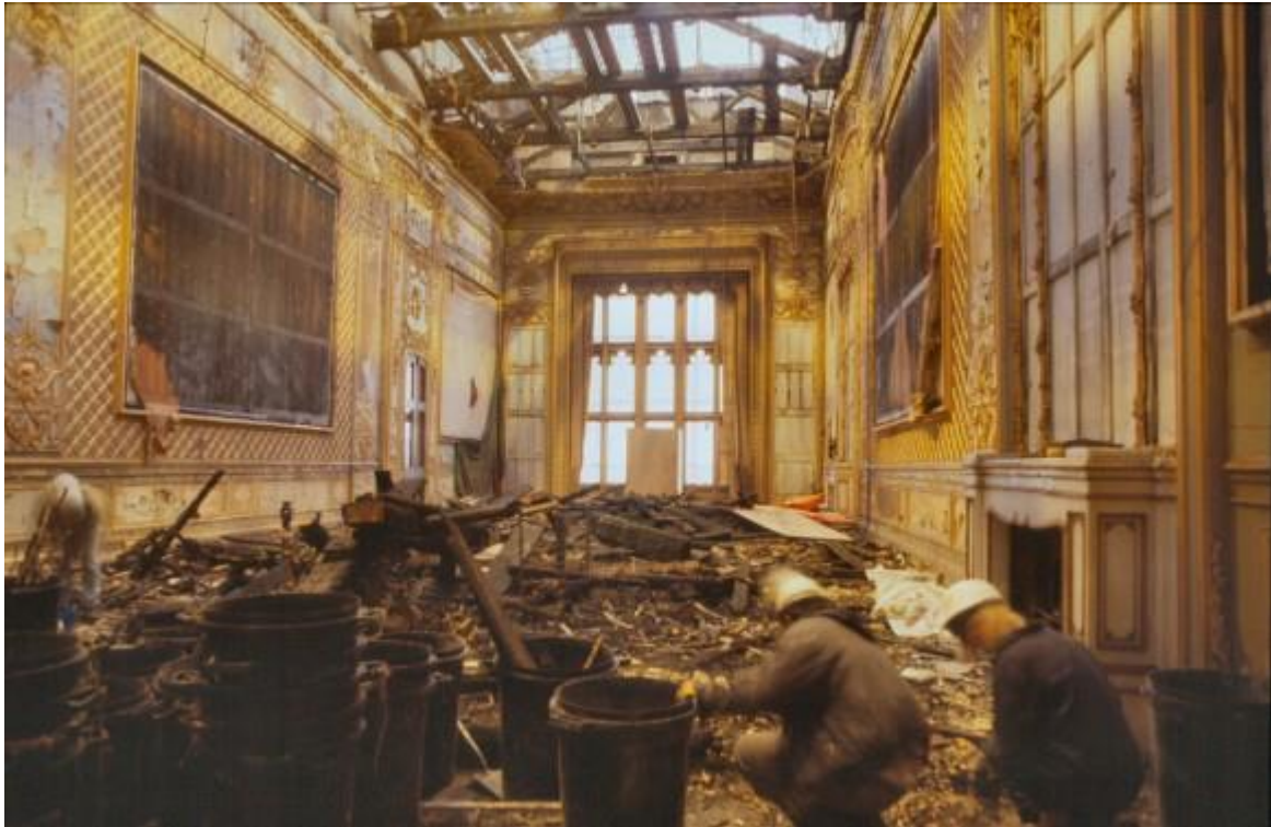
Archaeological salvage of fire debris starting in the Grand Reception Room, Windsor Castle, 1993
