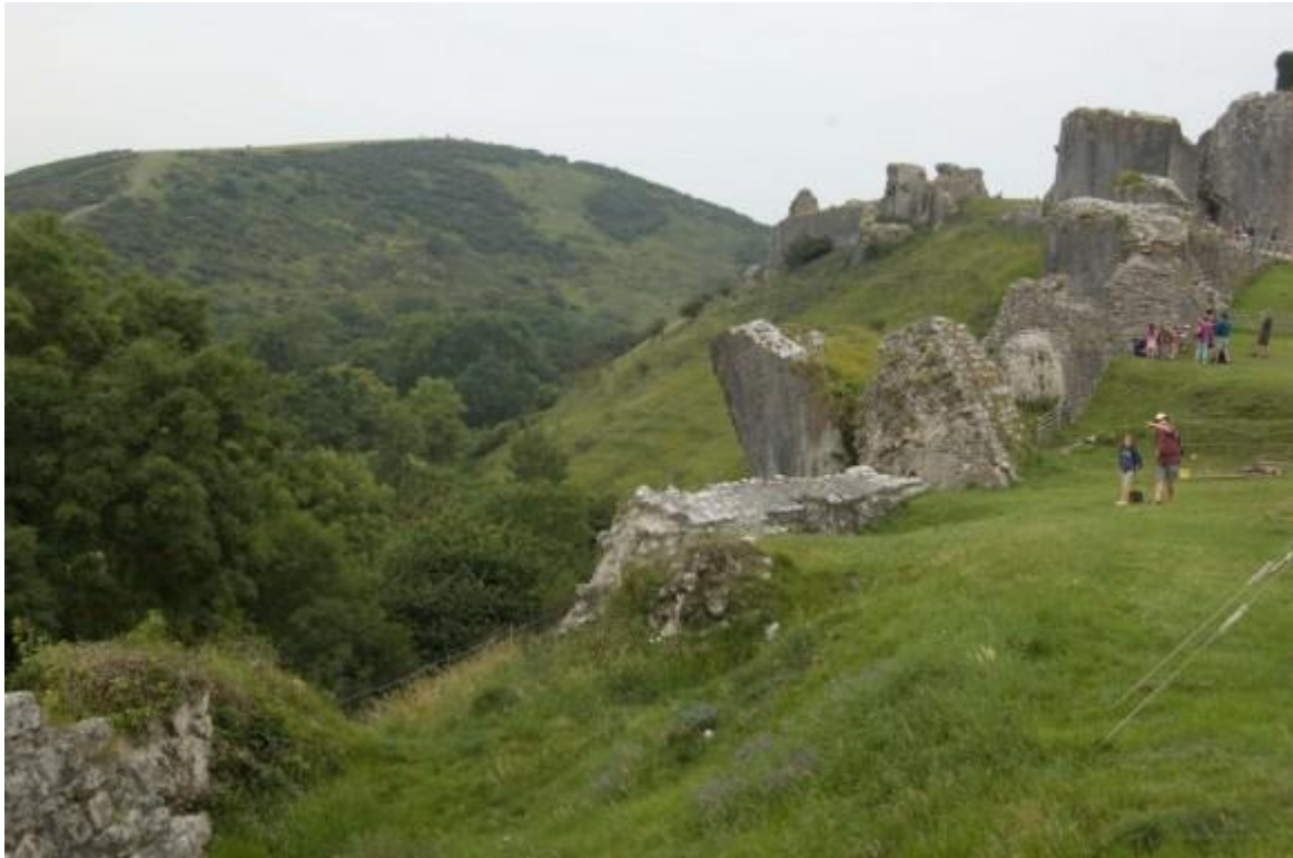
The effects of undermining - the tower has slid down the slope, and the curtain wall has fallen over.
