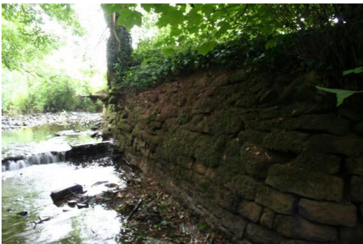
The structure curving away from the perpendicular
