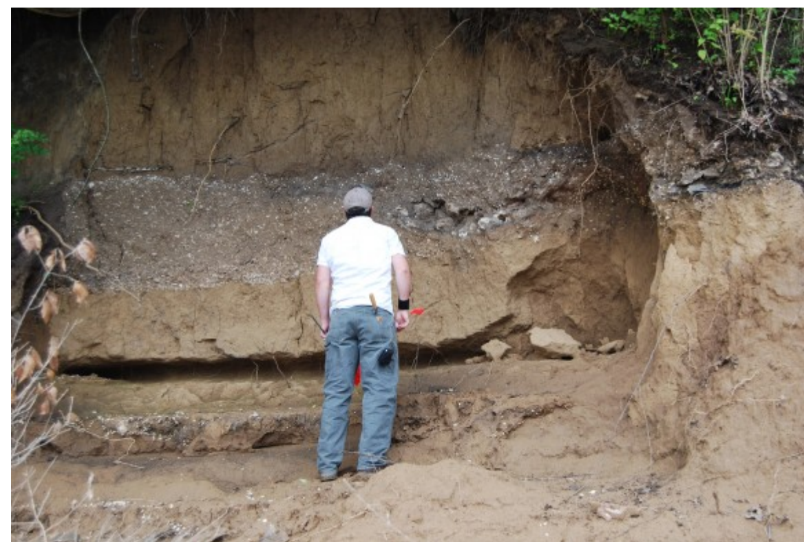
Site inspections along the riverbank.
