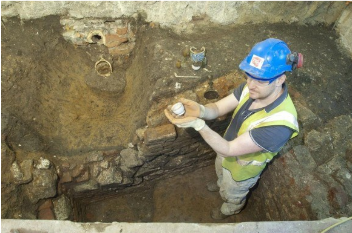
Andrew up to his elbows in an 18th century brick-lined cess pit
