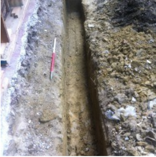
A slot foundation cut into very clean natural clay.
