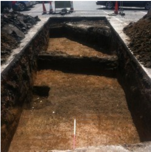
OK back to the trench. Very neat!
