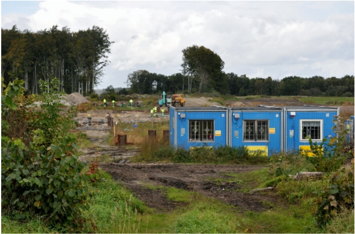
Excavation, Blekinge, Sweden 2011
