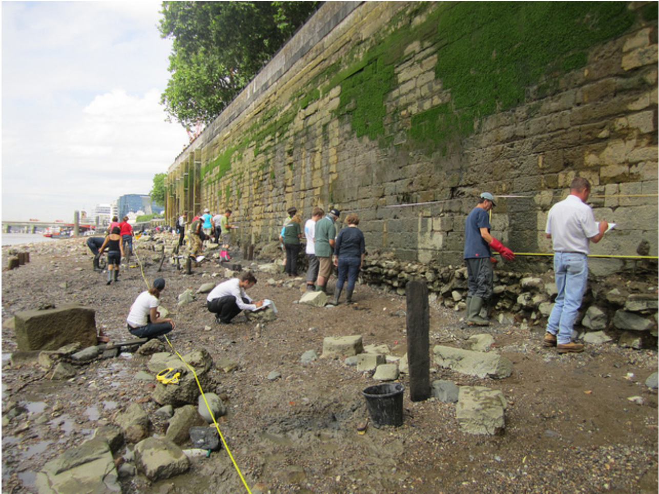
Recording the riverwall. The exposed foundations are at thigh height here.
