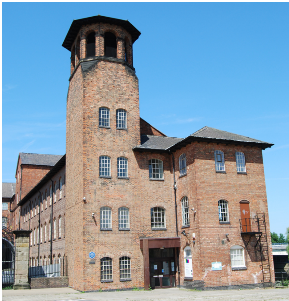
Derby Silk Mill (much rebuilt after early 20th century fire): one of the earliest factories in the world – part of the Derwent Valley Mills World Heritage Site
