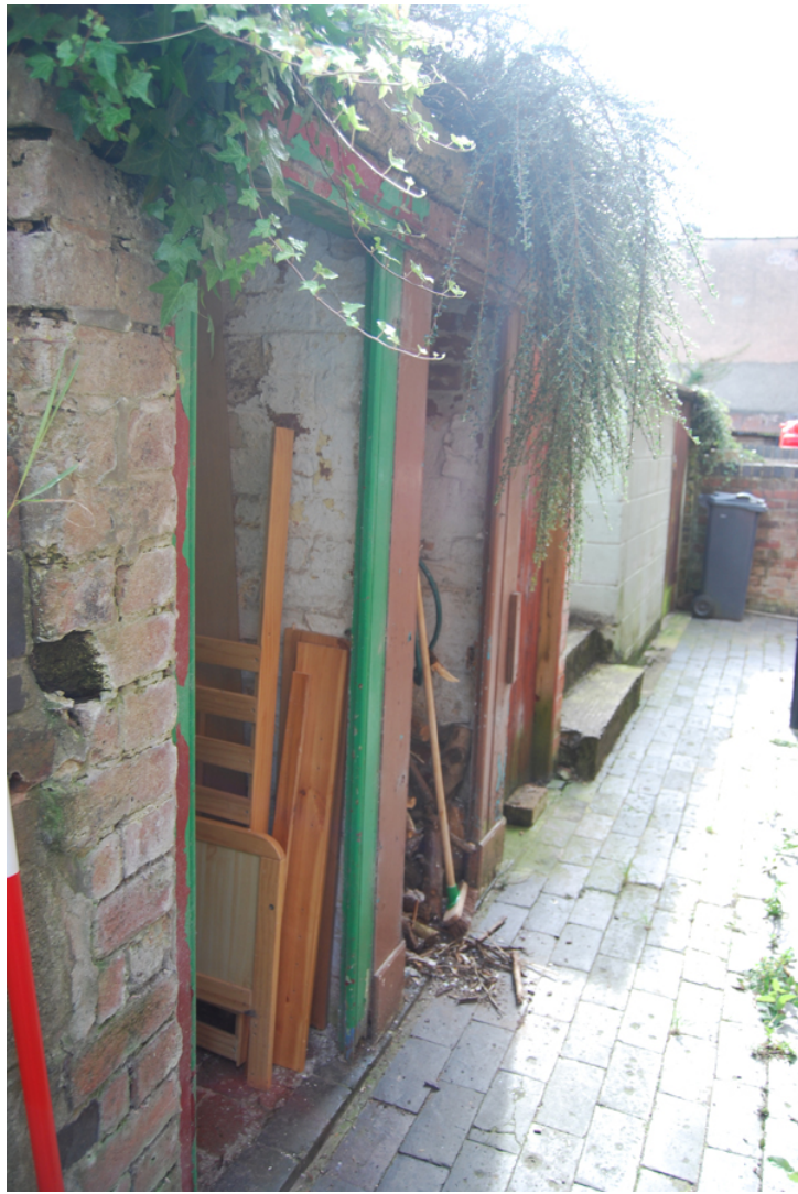
The remains of early toilets investigated at one property outside Derby
