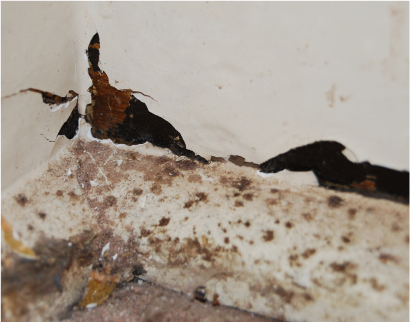
Chips to later white paint revealing remains of early finishes within LIPCAP case study: late 19th – early 20th century 'grained' varnish beneath dark early – mid 20th century paint, within project case study, No.
