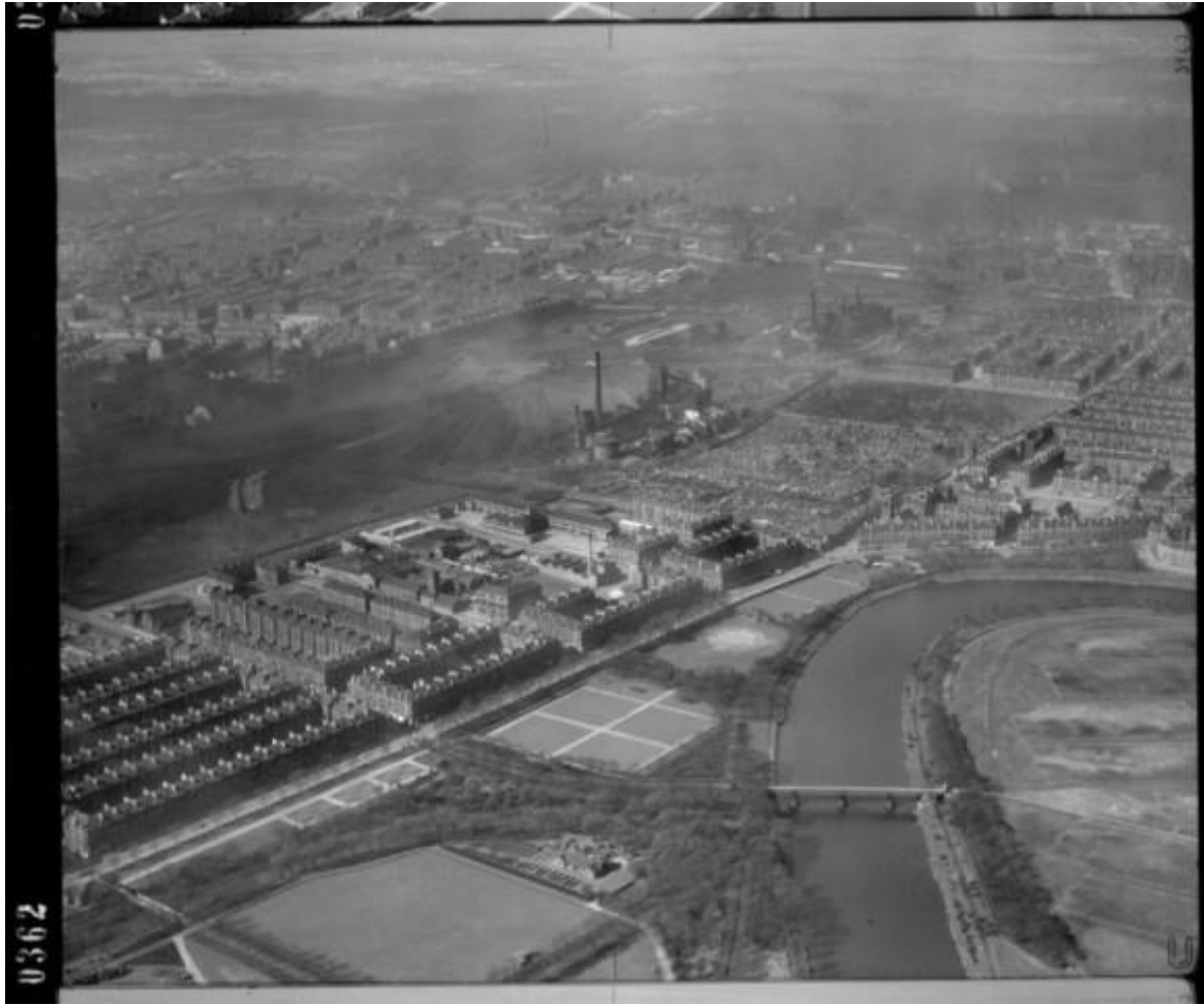
RAF National Survey (Air Photographs), 1944-1950 Scanned Image of RAF oblique aerial view showing part of the Hutchestown district with the Govan Ironworks (Dixon's Blazes) Copyright RCAHMS (SCI024381)
