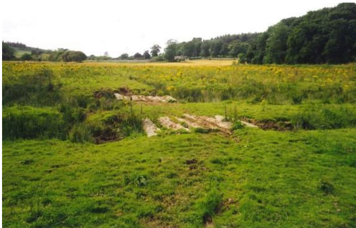
Two simple bridges at Mavisbank constructed of granite sleepers, providing access over the drains to the rigs. Copyright Iain Fraser
