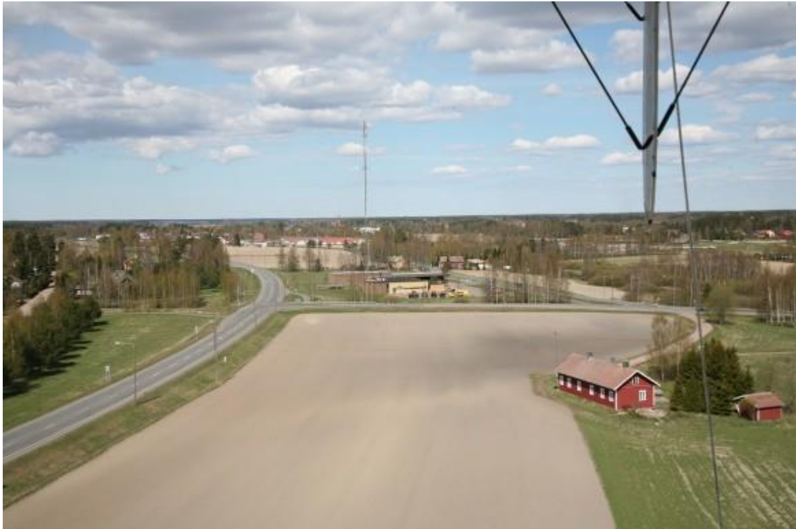
Low aerial photo from the excavation site
