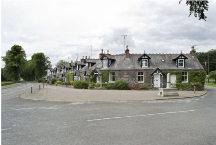
General view of Parton Village, taken from the ESE. Copyright RCAHMS (DP082914)
