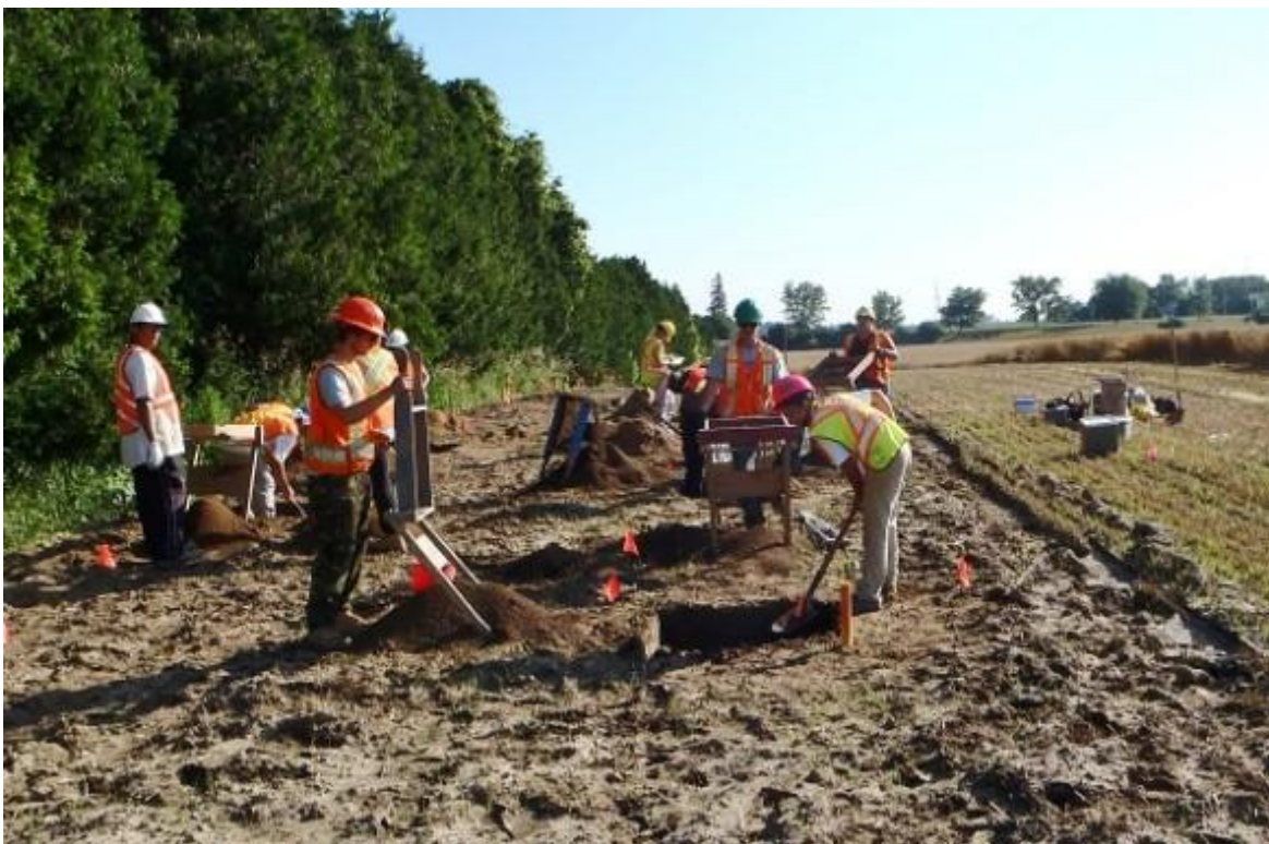
One of the crews excavating an area for the wind turbine project.
