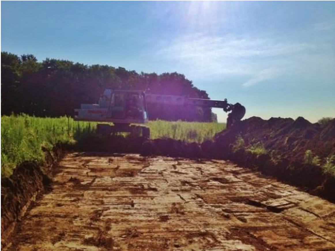
The Gradall machine stripping the topsoil off Robb's site.
