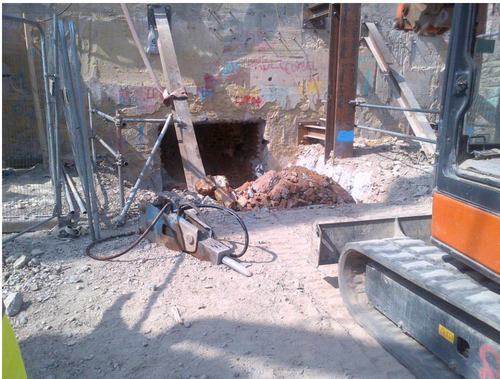
Start of the sewer heading (c) MOLA 2013
