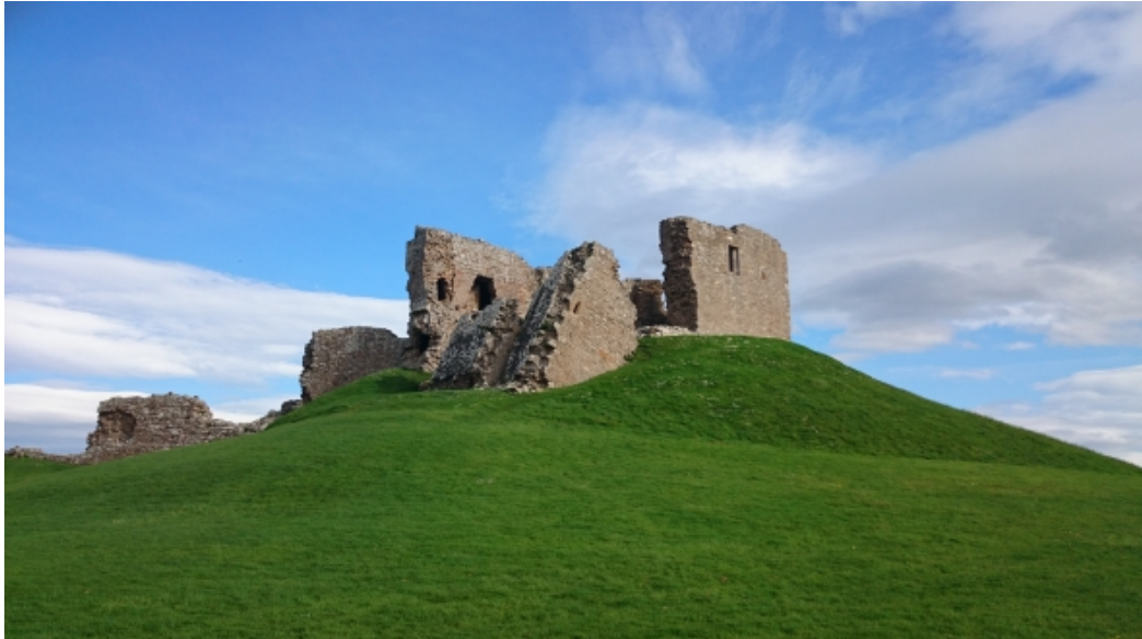
Duffus Castle, a motte and bailey castle in Moray. The timber castle on the motte was replaced with a stone keep in the 14th Century ©ACAS
