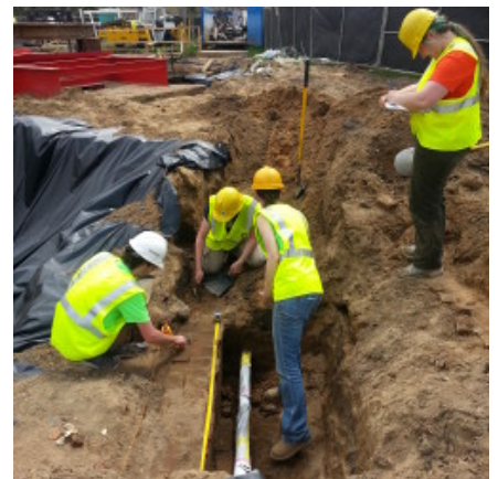
CAP crew excavating the west wall of the Old Vet Lab
