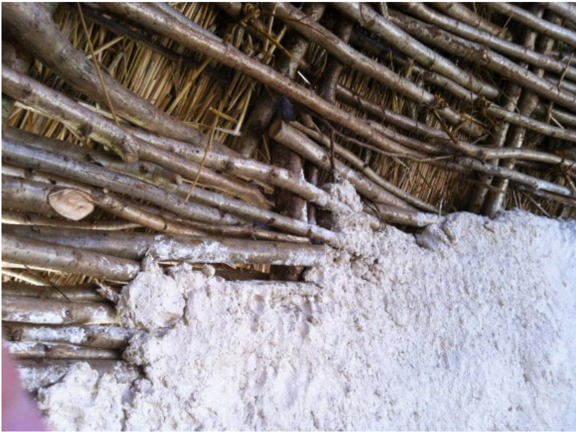
Putting the daub onto one of the Neolithic Houses
