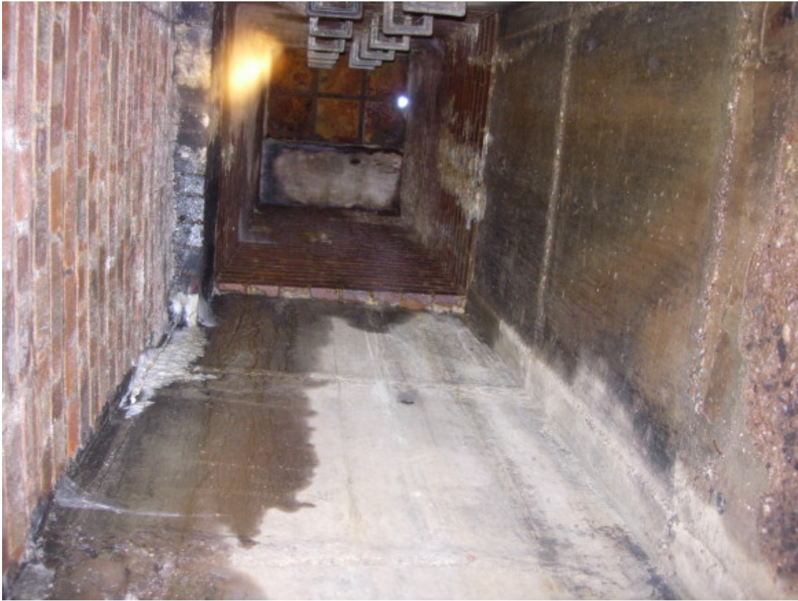
Metal ladder at east end of the tunnel
