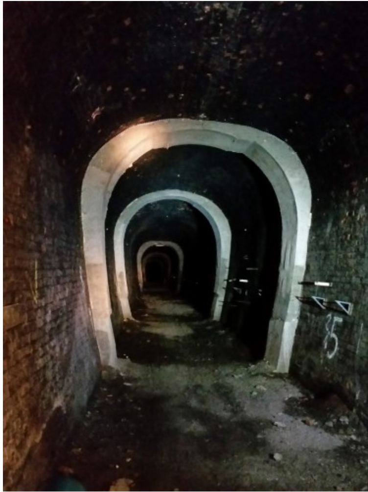
Concrete reinforcements inside the tunnel
