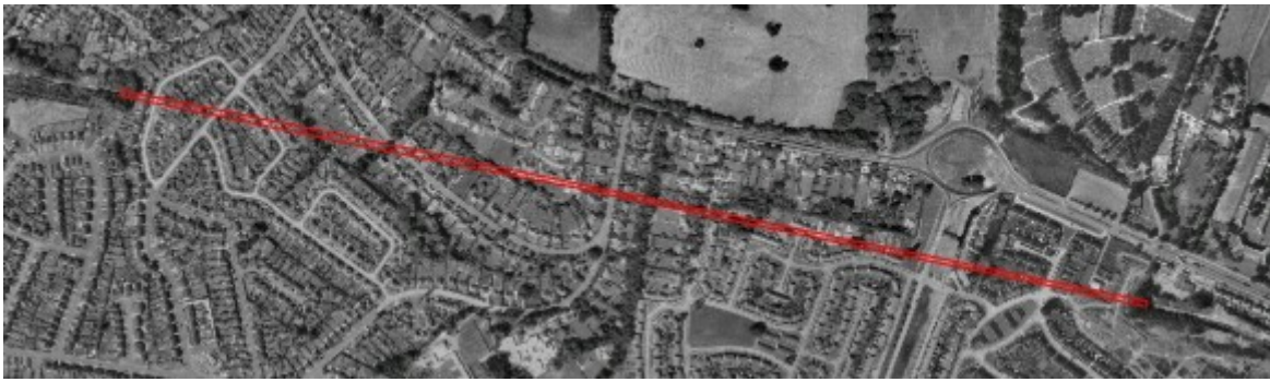
Glenfield Tunnel in 1969
