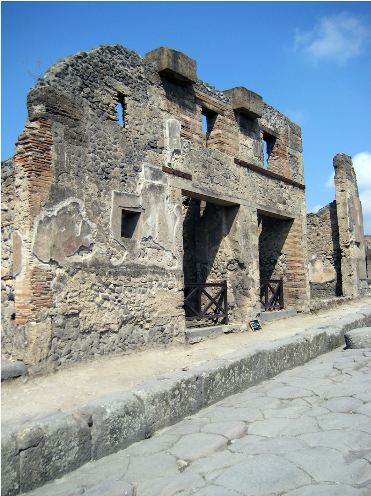
A bakery retrofitted into a two storey house (8.4.27), left, and a shop for bread (8.4.26), right. Another shop (8.4.25), far right. Copyright Sera Baker, 2016.
