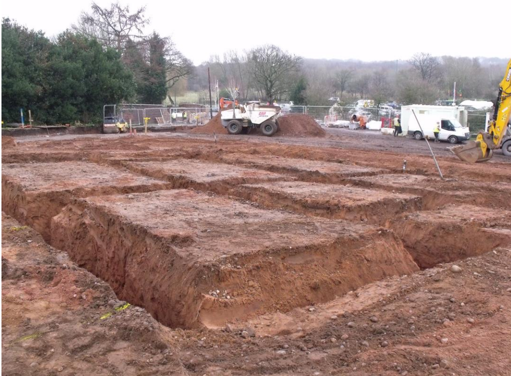
Plate 1: Construction foundation trenches showing extent of natural ground. Phase 1 area, Plot 1.
