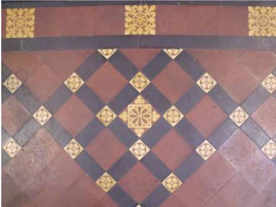
Plate 46: In situ tiles within St Giles Church (Godwin & Minton?) with the same designs to those of the recovered tiles, based upon their medieval counterparts.
