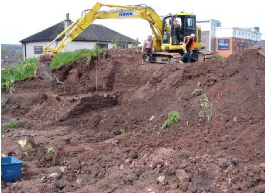
Plate 22: Spoil mound (1000) under excavation, facing north west.
