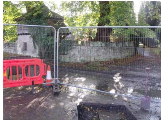
Plate 4— Drainage work in Church Close
