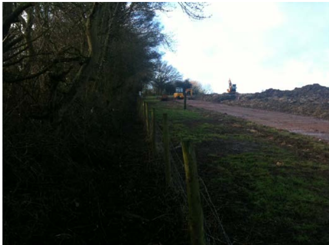
Appendix 5: Pre 1996 post and wire boundary fence, ditch and bank. 2012 facing west.
