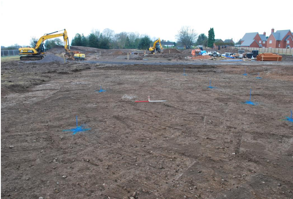
Plate 3: General view of construction area. 24 th January 2017. Facing south.
