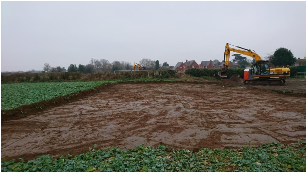
Plate 2: Detail of site compound excavation. 7 th December 2016. Looking south.
