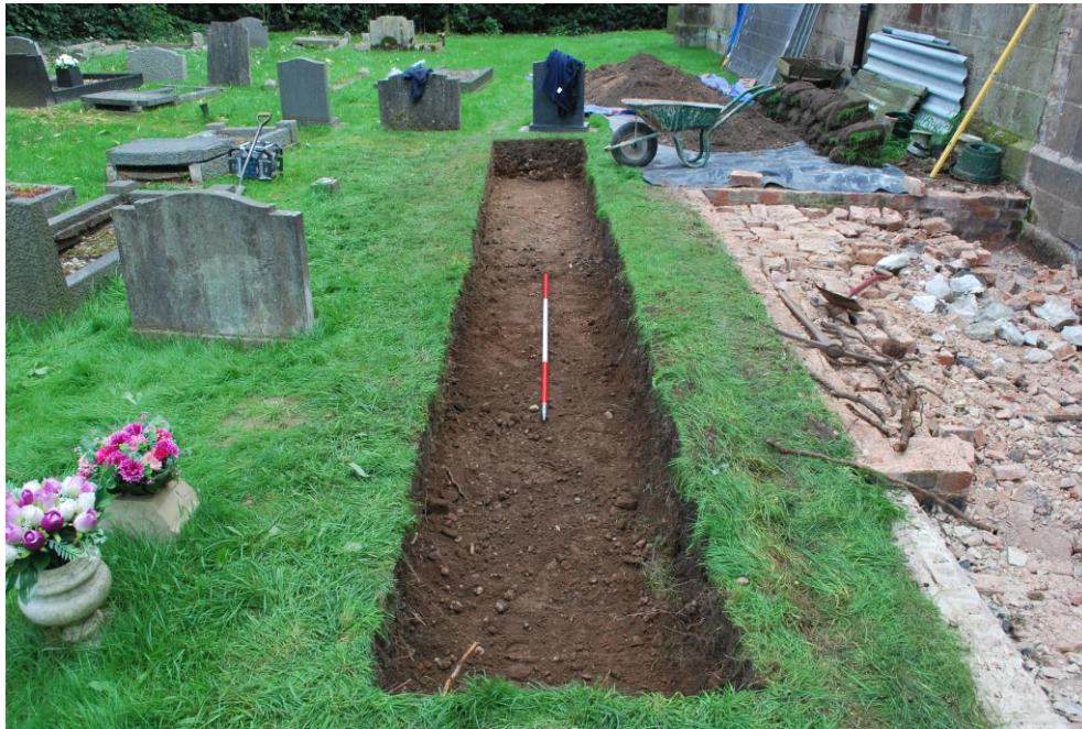
Plate 3. Foul water trench after excavation facing east
